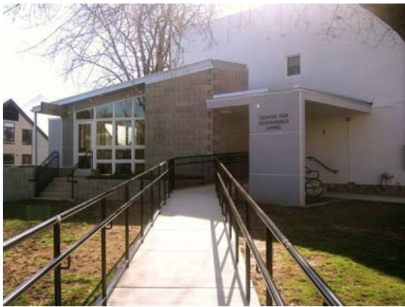
Photo: On Sun Mar 30th you can tour Dickinson’s Center for Sustainable living featuring grey water use, solar energy capture, low flow toilets and more.
